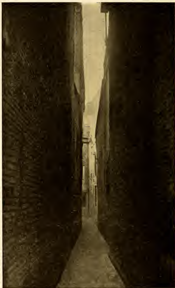
ALLEY LEADING FROM BARNESTEEG STRASSE
